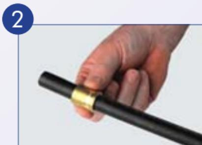
2 Slip the jointing sleeve over the end of the pipe with the beveled end of the sleeve facing outwards and the grooved end of the sleeve at the furthest point from the end of pipe.
