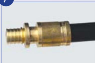
Inspect the joint to ensure the sleeves are drawn all the way to the fitting shoulder and the beveled end of the sleeves is towards the fitting.
